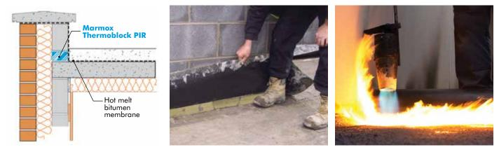
If applying a hot-melt bitumen membrane to a roof junction with a parapet wall using a flame torch, Marmox Thermoblock-PIR should be specified as this version is resistant to distortion which the standard block may experience if in contact with the flame gun. The PIR version has a slightly lower thermal conductivity (0.041W/mK), is 53mm high and like the standard version a compressive strength of 9N/mm<sup>2</sup>.
